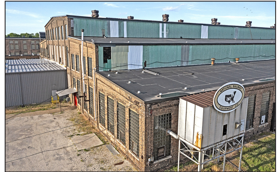
A National Railway Equipment Company sign is on the southwest corner of former Chicago, Rock Island & Pacific Railroad Silvis Shops erecting shop at Silvis, Illinois, on June 9, 2022. National Railway Equipment sold the buildings to Railroading Heritage of Midwest America in May 2022. – Photo © 2022 by Chip.
